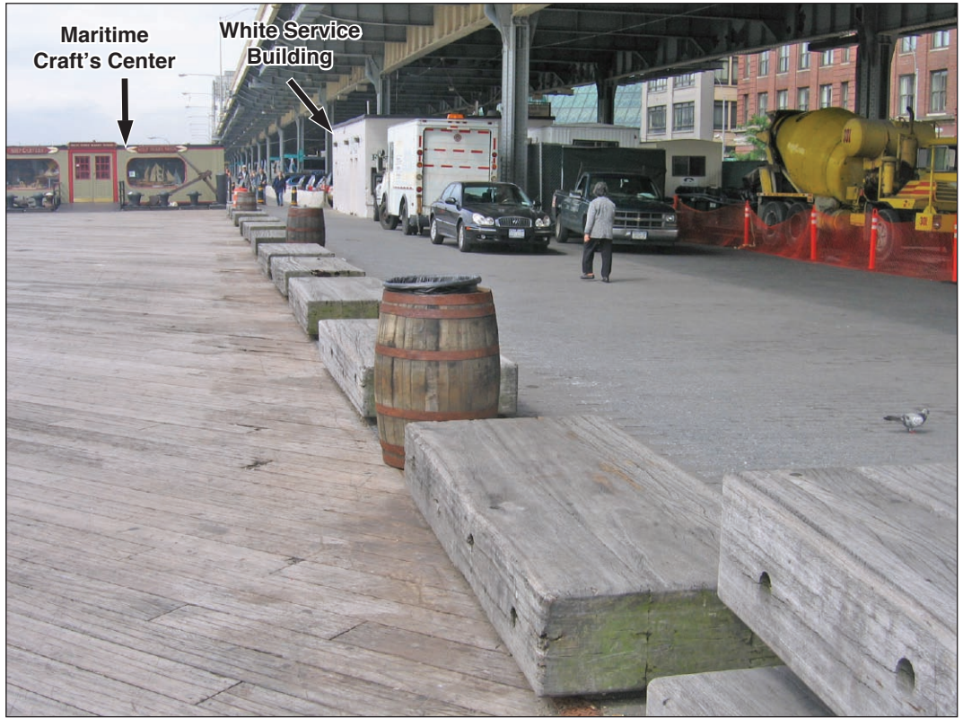
View south from near Pier 16 2
