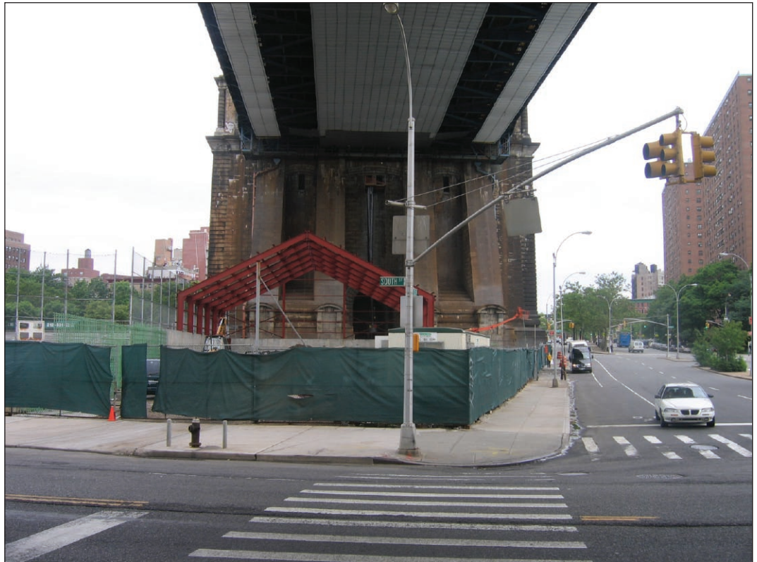
Manhattan Bridge pier 46
