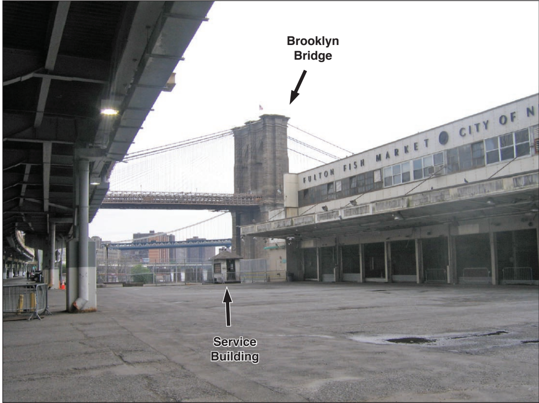
New Market Building (former Fulton Fish Market Building) 3
