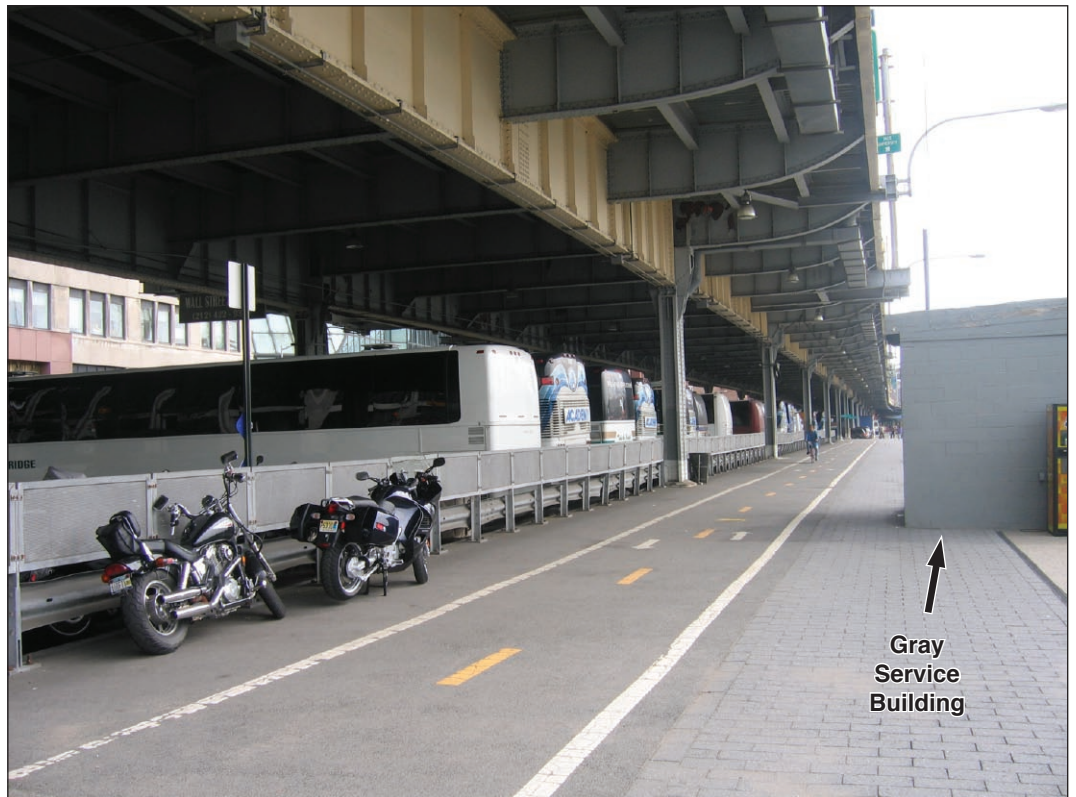
View north from near Pier 13 20
