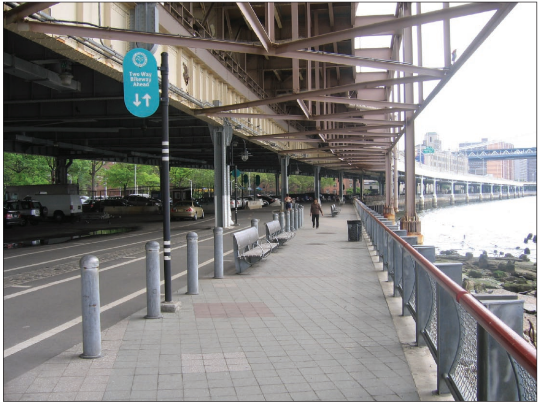
FDR Drive cantilevering over the esplanade and the East River 21
