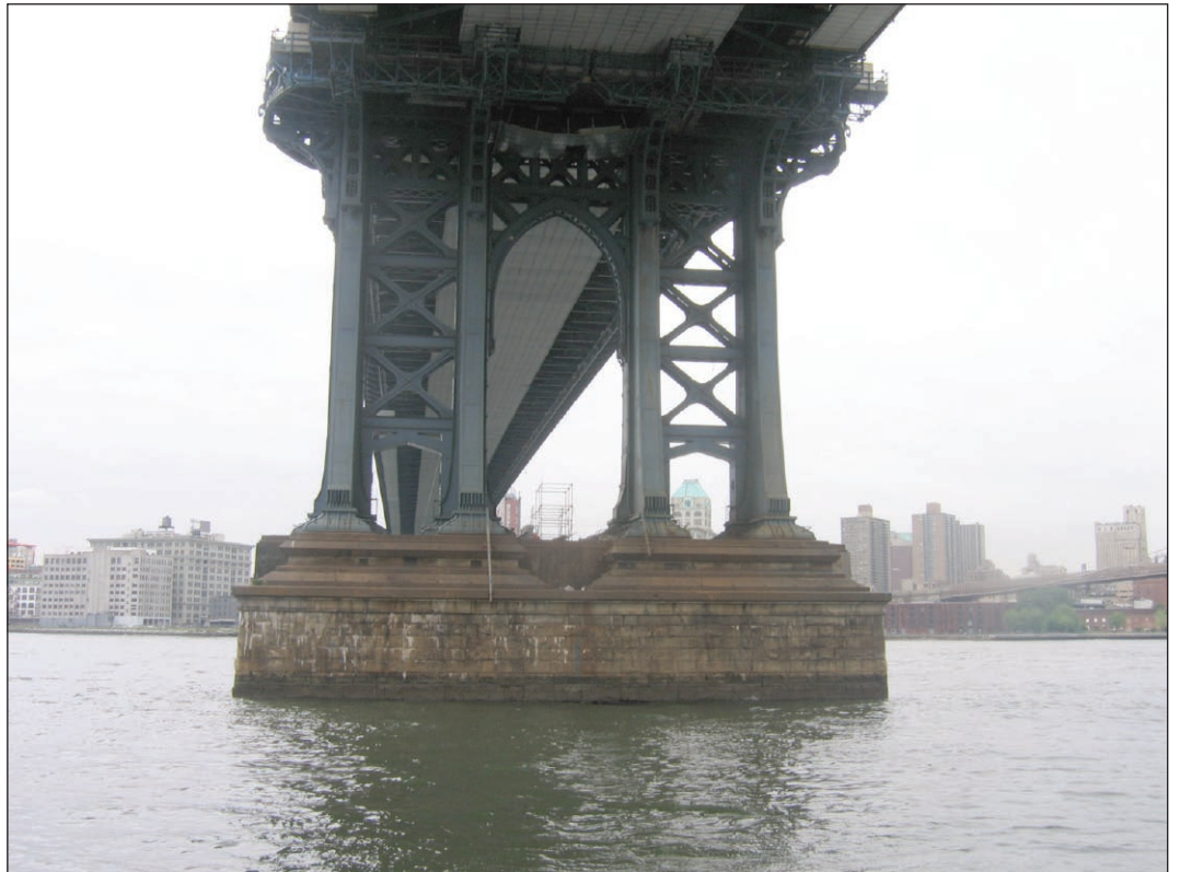
Manhattan Bridge Pier 53
