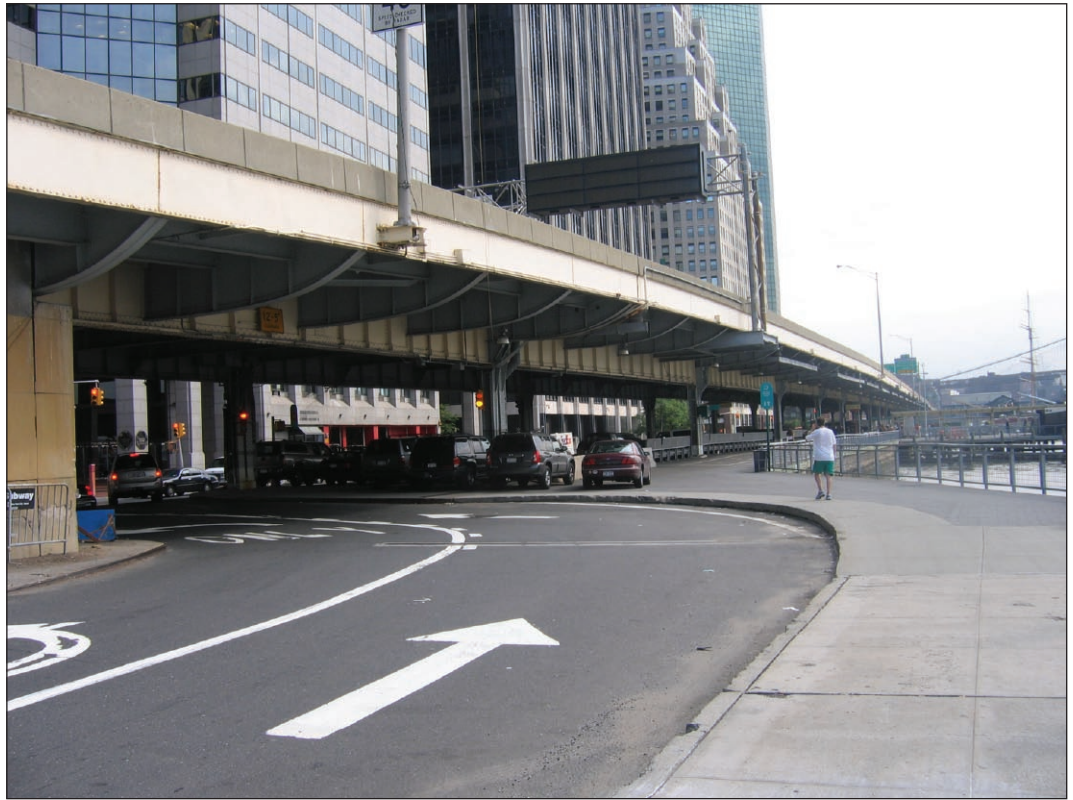
View north of the FDR Drive from Old Slip 10
