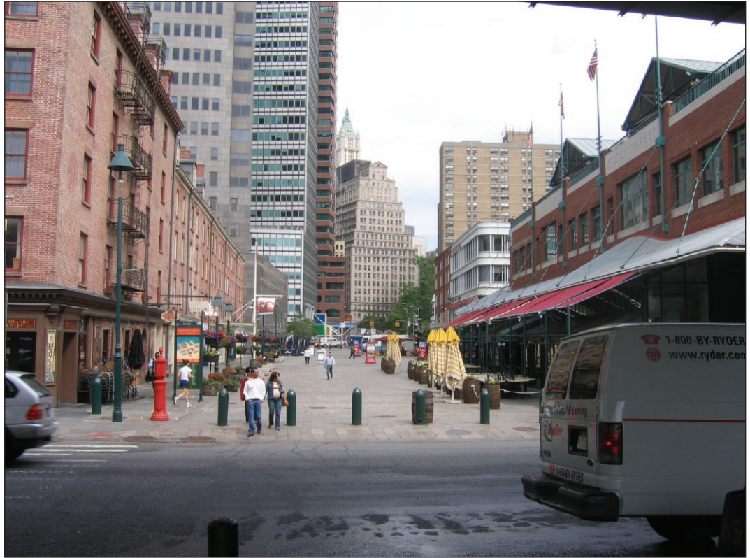
Fulton Street view corridor 32
