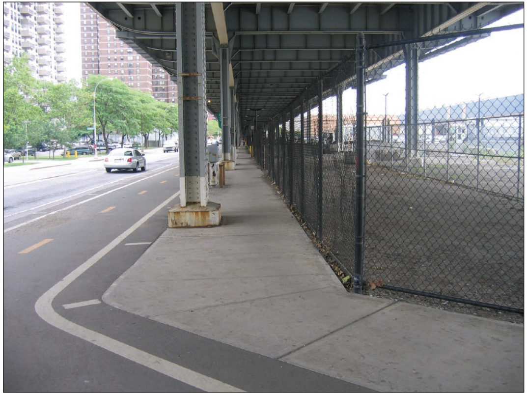
View north of the walkway/ bikeway north of Pier 35 23
