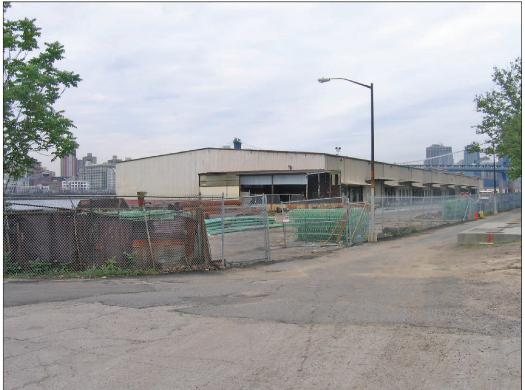
View from the north of Pier 42 5
