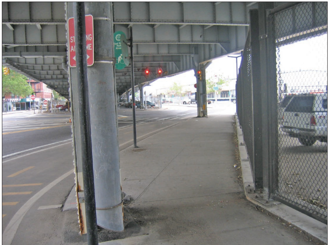
Northern end of the walkway/ bikeway at Montgomery Street 24
