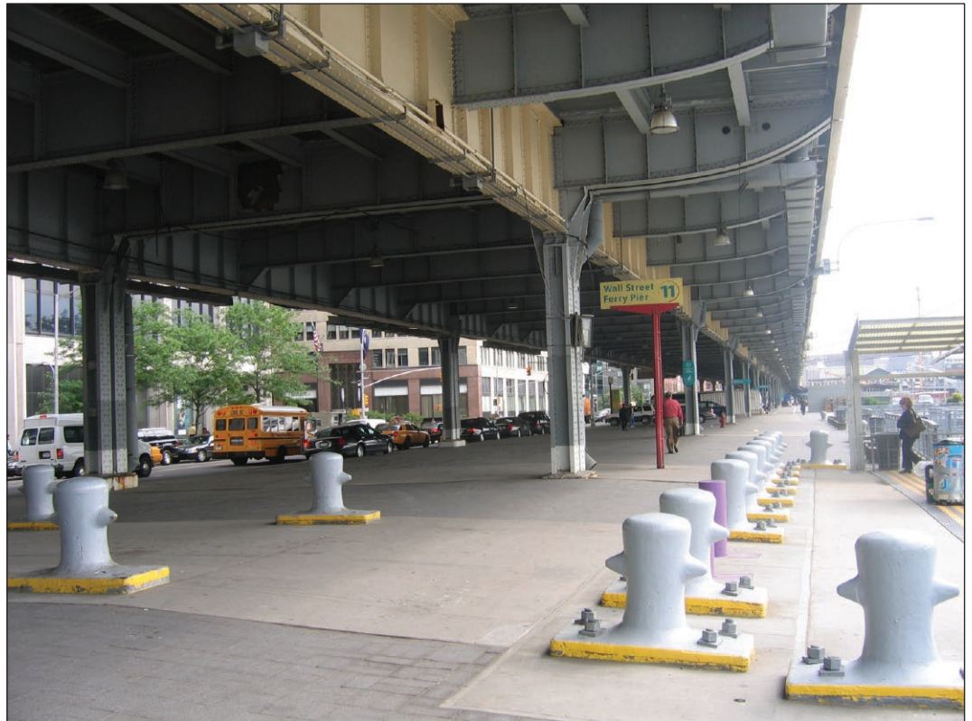
View north from near Pier 11 19
